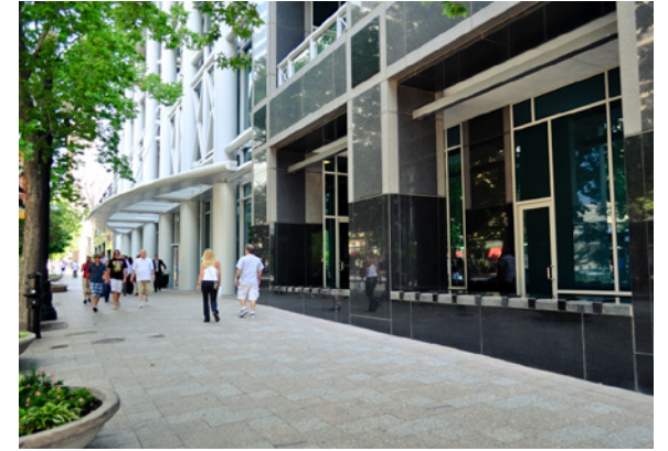
Skyscraper with Poor Visual Permeability on Ground Floor
