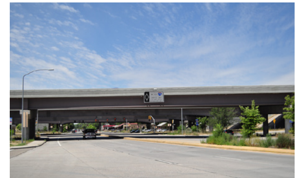
400 South (Looking West)
