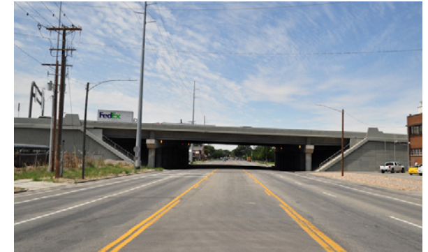
800 South (Looking West)
